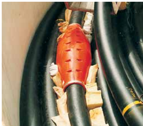
Flange Protector on flexible pipe.
