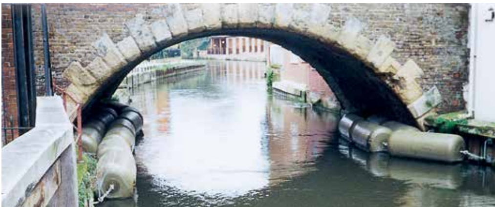
Canal bridge protection.
