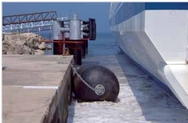
Type II fender in operation
